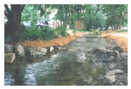
Water Street After: Rock structures were placed to narrow the stream channel, improve aquatic habitat and give high water better access to floodplain
