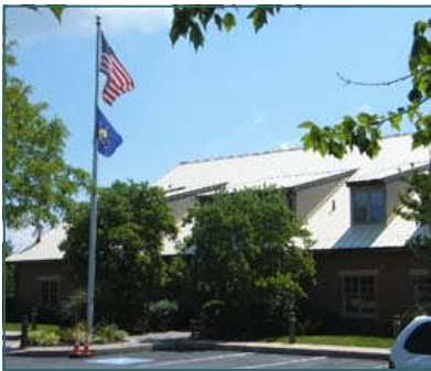
Pictured above is the new "cool roof" on the Warwick Township Municipal Building
